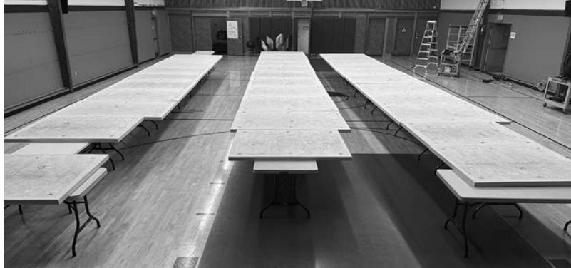
Laying out all the panels before installation.
